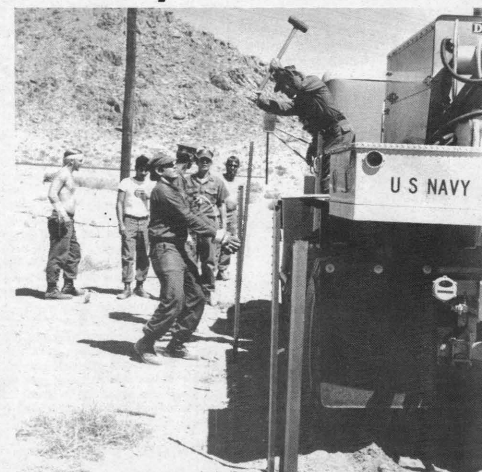
VITAL WORK — Tackling the difficult assignment of installing perimeter security fencing around NWC were these personnel from Detachment 0217 and the Seabee Self-Help unit at China Lake. In the photo, the Seabee with the sledgehammer is standing on a welding truck as it accompanies a work party near the sewage treatment plant.
