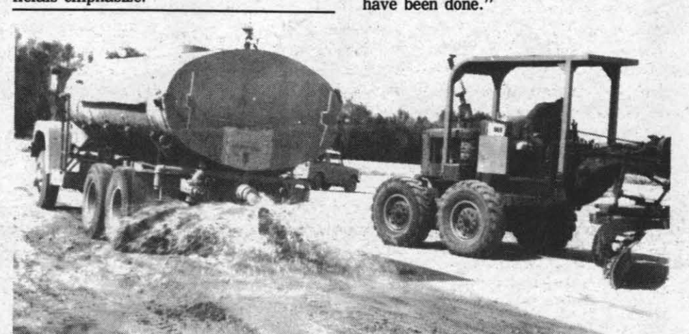
FOR SAFETY'S SAKE — One of the many popular projects on-Center undertaken by the Seabees was construction of bike paths, like this one pictured near Burroughs High School. In the photo, the water truck's job was to settle the earth for later grading by the machine at the right. —Photo by Ron Allen
