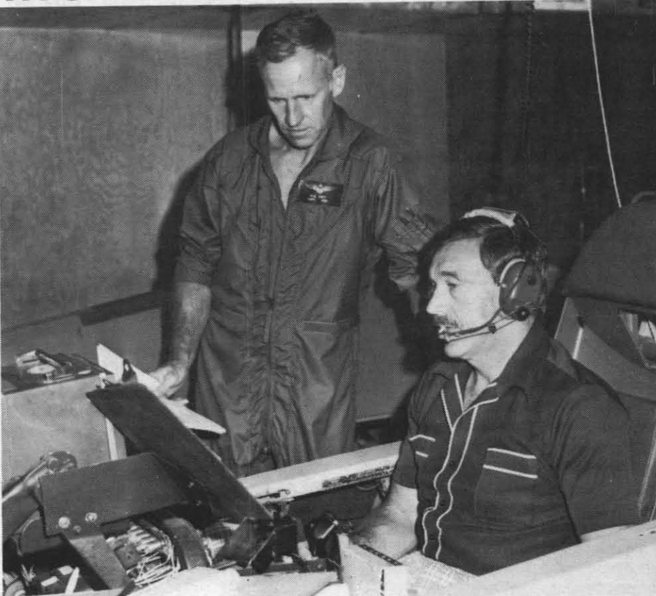
DEAN OF NOLO AIRCRAFT FLIGHTS — With Capt. W. B. Haaf, NWC Technical Officer, looking on, Harlan Reep goes through a simulation of the various operations involved in piloting a drone aircraft from the Naval Air Facility Targets Department's remote control ground station. —Photo by Ron Allen
