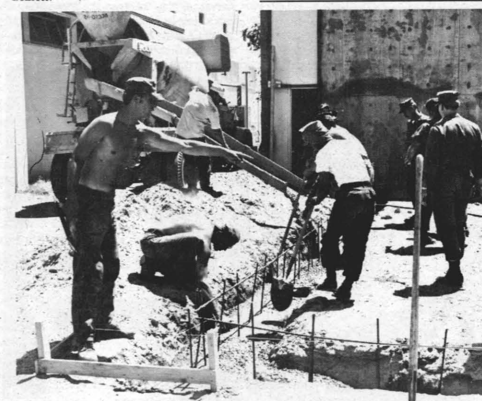
HANDBALL COURT FOUNDATION POURED — Members of the Naval Mobile Construction Battalion 40, from Port Hueneme, spent a week at the Naval Weapons Center working on different Self-Help projects, including the pouring of the foundation for the new handball court at the Center gymnasium (above). This task was headed by BU1 Richard Peters (at left). —Photo by Ron Allen
