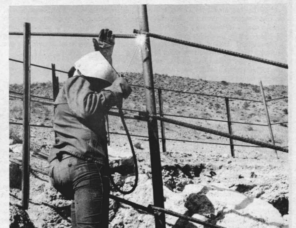
BURRO BARRIER — Fencing around the natural springs at Layton Canyon and Amity Springs was erected to prevent wild burros from digging down for water and clogging up the springs. SW1 Randy Matt was one of the Seabees who handled the hot job of welding sections of the structural steel fence together.
