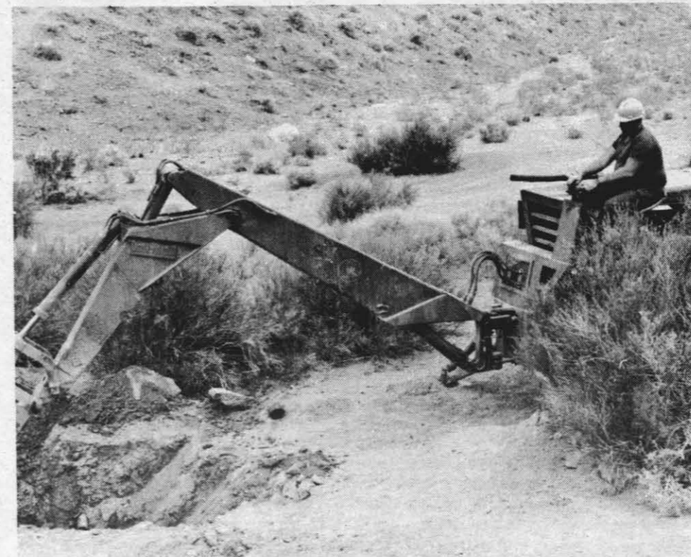
PIPELINE TRENCH DUG — Using a back hoe, EO2 Art Pankey digs a trench in preparation for laying pipeline from a spring in Layton Canyon to a large trough that will collect water for consumption by wild burros in the area.
