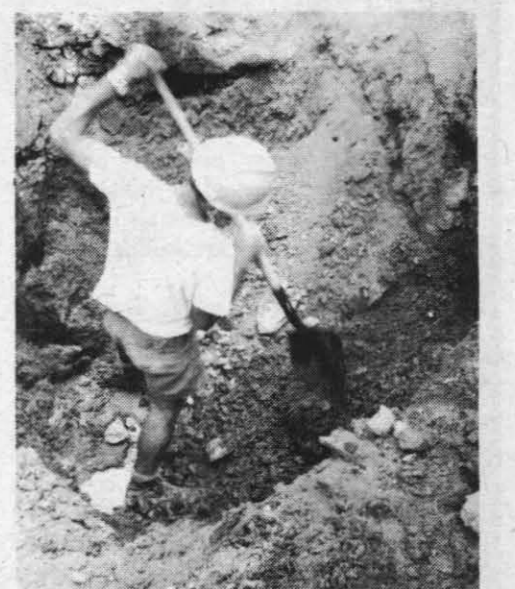
HOT WORK — It didn't take long to work up a sweat while using a shovel to clean out a water seep that feeds Amity Spring. Shown above doing just that is SWC Bob Reagan, assistant officer-in-charge of Seabee Team 1024.
