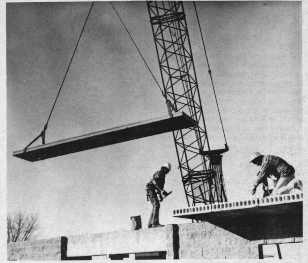
SECOND DECK FLOORING INSTALLED — A huge crane has been used this past week for lowering into place the pre-stressed concrete planks that form the second deck of the new Bachelor Enlisted Quarters (BEQ). The planks are pre-fabricated from tensioned cables and concrete prior to delivery to the job site. Their use provides substantial savings in construction costs. While this work has been under way on the first of three separate BEQ quadrangle complexes, masonry work also has been started on the first-story walls of the second quadrangle and, at the same time, electrical and plumbing work is continuing. Masonry work on the second story of the first building will be resumed as soon as the second deck is in place. —Photo by Ron Allen
