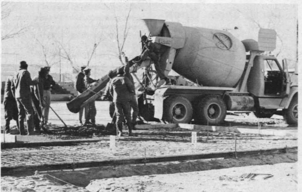
SELF-HELP PROJECT AT NAF - One of the many Self-Help projects worked on during the past two years that helped NWC win the 11th ND Bronze Hammer nomination, was the improvement of the NAF swimming pool and recreation area.
