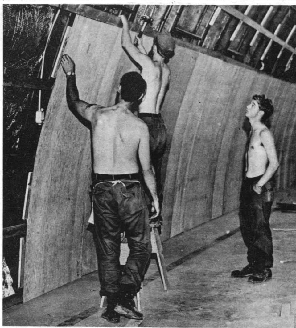
SEABEES LEND HELPING HAND — Looking ahead to the coming basketball season, when there will be heavy pressure on the use of the Center gym, preparations are going ahead to convert the former Shopping Bag annex into a youth gym. As part of a Self-Help project, a group of 10 Seabees from the U.S. Naval Support Force Antarctica spent the past two weeks here installing plywood sheeting to form the interior walls of the new youth gym facility. The visiting Seabees also added onto the block wall being erected at the site of a mobile home park for military personnel located on Princeton St.
