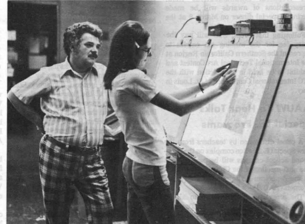
EXACTLY RIGHT — Jack Lindsey supervises layouts of the paper each Thursday afternoon. Here, Phyllis Orr (who is no longer employed at The Daily Independent) lays in a "window" on the paste-up page. A window is a red piece of paper that photographs as clear as a page negative, allowing the stripper to place a photo negative on top of it.
