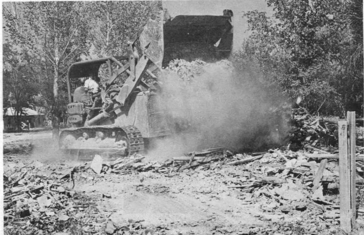
DEMOLITION WORK UNDER WAY — This is the fate of 27 more old Hawthorne-type housing units located on Princeton and Ranger Sts. Tearing down the old structures and clearing away the remains, a job that is scheduled for completion by mid-November, is being handled by workmen for the Aiden Slaybaugh Demolition and Trucking Co. under a contract totalling $17,280.
