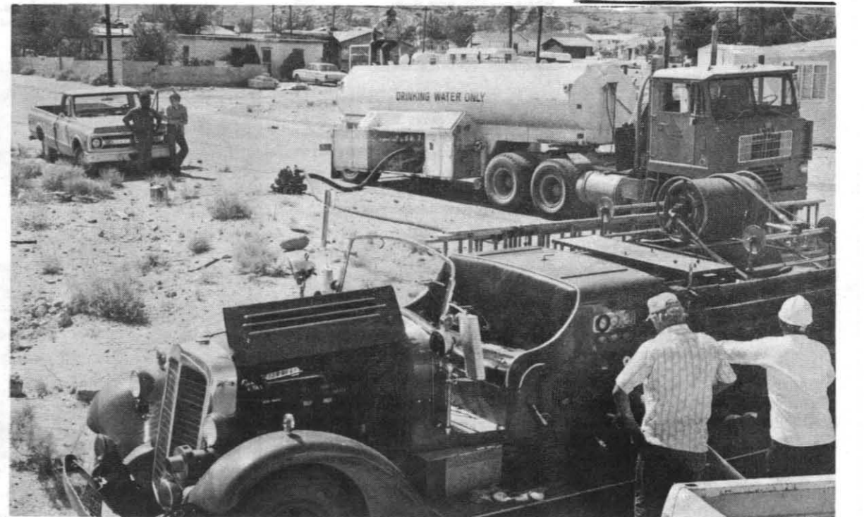
EMERGENCY AID PROVIDED - A helping hand in alleviating a water supply problem was provided last Friday by the Naval Weapons Center in the Pioneer Point area of Searles Valley. Water hauled by the Navy tanker truck (in background) was drawn into a fire department pumper truck and from it forced under pressure uphill into a nearly dry storage tank. -Photo by PHAN Jerry Sizemore
