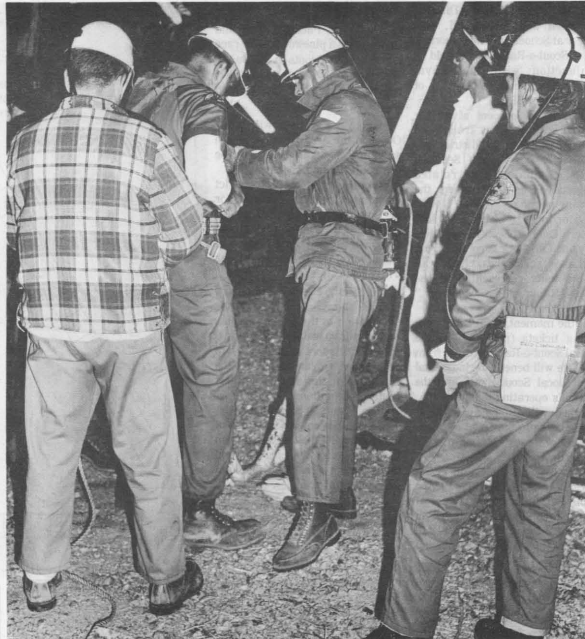
AFTER A CHECK by Camphausen (right foreground), Bob Wilhelm is "suited-up" for a descent into the shaft. Jack Williams is fitting a harness on Wilhelm to which the three lines are attached.
