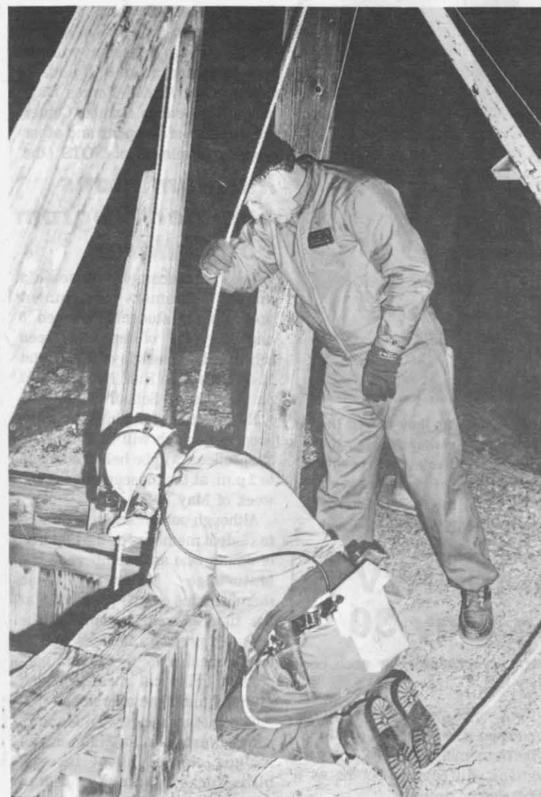
SAM WYATT (standing) team captain, observes the clearance of the three lines used when hoisting a man up or down in the shaft. (They are the main hoist line, a safety line, and a telephone line.) The man kneeling, watching Camphausen's progress, is Bob Padgett.
