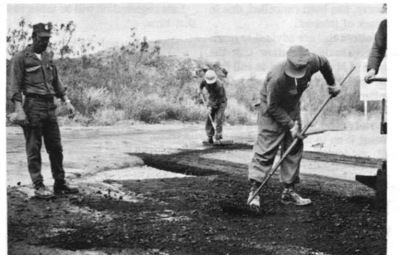
MUCH PAVING DONE — Men of MCB 17 spread asphalt for a road in front of the Marine barracks at Roosevelt Roads NAS, Puerto Rico. Six heavy equipment operators from Seabee Reserve Sub-unit 11-2, based at China Lake, were utilized on this job, as well as in work on a 2,500 yd. cutoff road at the Puerto Rican Naval Base.
