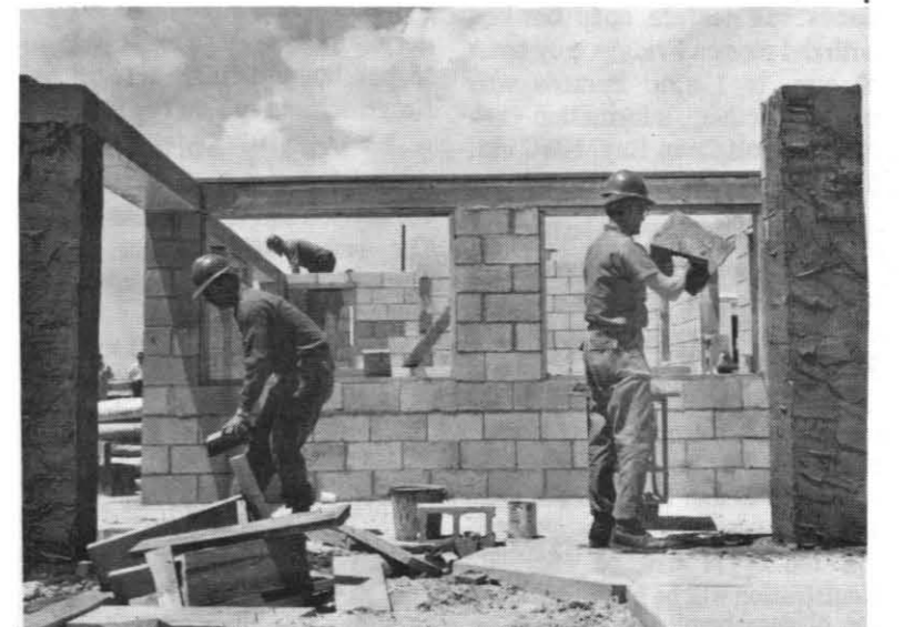
CPO CLUB ADDITION — Jim Stevens, of the local Sub-unit 11-2 of Reserve Naval Mobile Construction Battalion 17, was placed in charge of the building of a beach house addition to the Roosevelt Roads NAS Chief Petty Officers' Club. Above, workmen take advantage of the Puerto Rican sunshine as they work on the addition.
