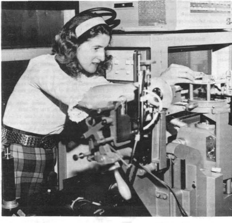
JEAN BENNETT adjusts the interferometer to obtain sharp FECC interference fringes of a mirror surface. These fringes contour the micro-irregularities on a surface, and show details only a small fraction of a wavelength in size.
