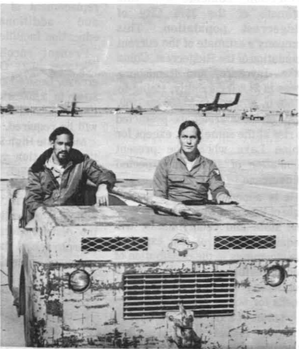
ADR3 D. R. Jones and ADJ1 Charles Malear (left and right, respectively) operate a tow truck, which pulls aircraft to parking positions on the apron.
