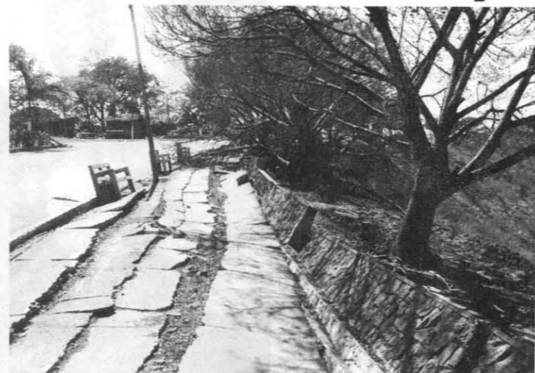
TYPICAL DAMAGE — A landslide along the edge of the Tescapa crater, around which the City of Managua is built, left this scene of damage following the destructive earthquake of last Dec. 23. Not far from where this picture was taken are the Nicaraguan presidential palace and the U.S. embassy — both of which were a total loss. The direction the trees are leaning indicates that the land in this area slid to the right, it was noted by Dr. Pierre St. Amand, who snapped the photo.
