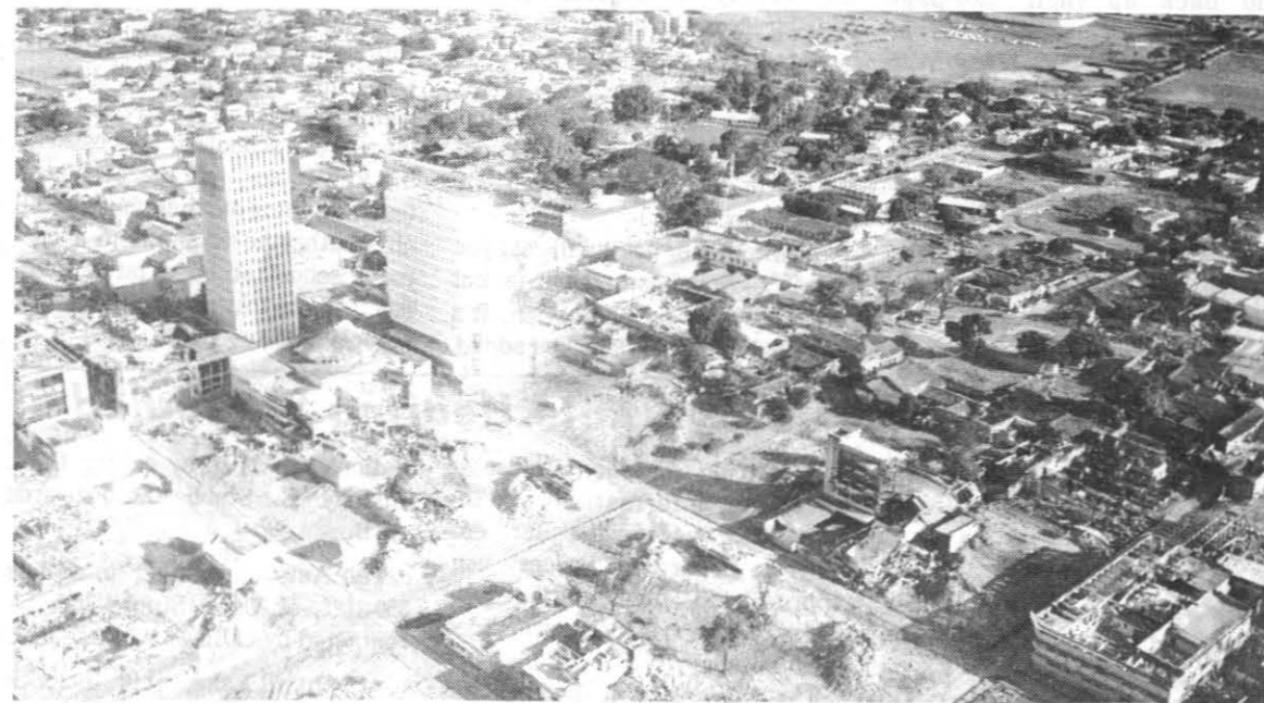
EARTHQUAKE BATTERED CITY — This aerial view of the badly damaged City of Managua was snapped by Dr. Pierre St. Amand while riding as a passenger in a Cessna aircraft being flown by a Nicaraguan Air Force pilot. The two taller structures (both bank buildings 15 and 20 stories high) bear out Dr. St. Amand's contention that well-constructed buildings can withstand earthquakes of the type that flattened most of Nicaragua's capital city. The NWC scientist found that a gravel mat under the taller of the two buildings had insulated it against the Dec. 23 earthquake which brought near-total destruction to the downtown area of Managua. When this photo was taken, demolition work had already been started and the debris from a number of demolished buildings hauled away.
