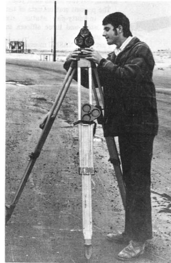
BILL KINGSLEY (left), a Co-op student from the New Mexico State University, at Las Cruces, adjusts the mirror lenses on his surveying gear, while in the right photo Jan Gieger (left), and Butch Lamson send an infra-red signal to Kingsley's apparatus. What they are using is a precision instrument that measures distances by infra-red signals to perform surveys. The equipment is accurate to 1/2 centimeter over a two-mile distance.
