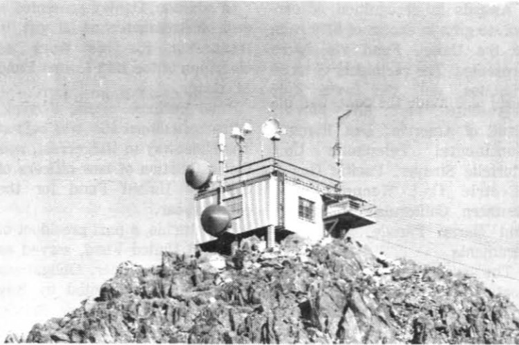
THIS FREQUENCY monitoring station is located south of the Instrumentation Lab, on top of the Lark Ramp, and is 20x20ft. Inside is a myriad of monitoring equipment.
