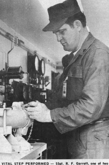
Marine staff NCOs trained to operate the missile maintenance van, practices one of the key operations--recharging of the Sidewinder launcher gas receiver.
