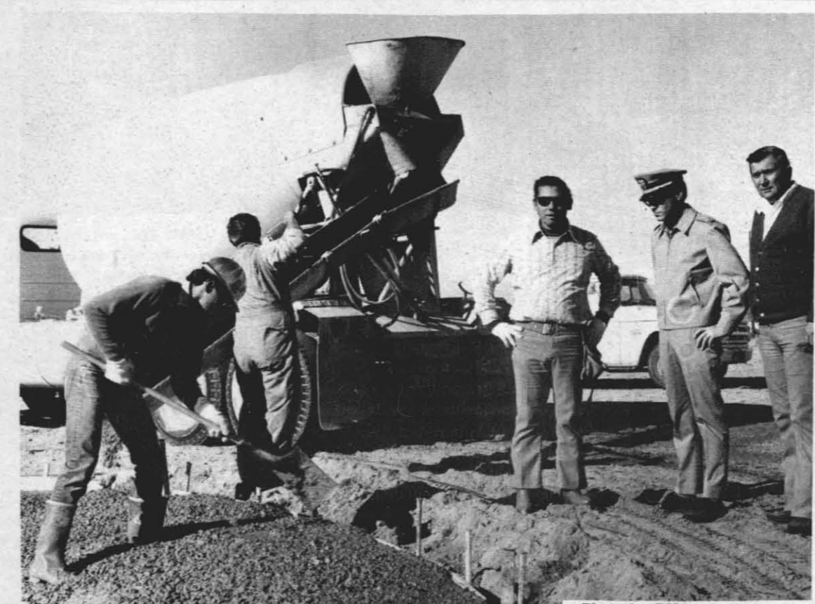
EMERGENCY HELIPORT CONSTRUCTED—Following up on grading and site preparation work that was handled earlier by members of Reserve Naval Mobile Construction Battalion Sub-unit 11-2 of China Lake, concrete was poured last Saturday for the landing pad of an emergency heliport to serve the Ridgecrest Community Hospital. The landing pad, 25 ft. in diameter and up to 8 in. thick in the center, is located on Navy land across China Lake Blvd. from the hospital entrance. Looking on as the work began Saturday morning are (l.-r.) John Enriquez, of the S&E Construction Co. in Bakersfield; Ens. L.S. Murphy, project officer in the NWC Public Works Department, and Jake Gaddis, of the Ridgecrest Concrete Co. Enriquez brought a 5-man crew here to perform the labor, free of charge, while Gaddis' firm supplied the concrete at cost to the Rotary Club of China Lake, local service club whose members saw the need and contacted the necessary authorities in order to bring about this development. NWC's Public Works Department, headed by Capt. W. H. Sturman, played an important role in assisting the Seabee Reserves and clearing the way for obtaining permission to build the heliport. Yet to be completed is the building of a sidewalk and the installation of a fence around the heliporter landing pad. In the event of an emergency, however, the heliport could be used as it now exists. —Photo by PHAA S. K. Borders
