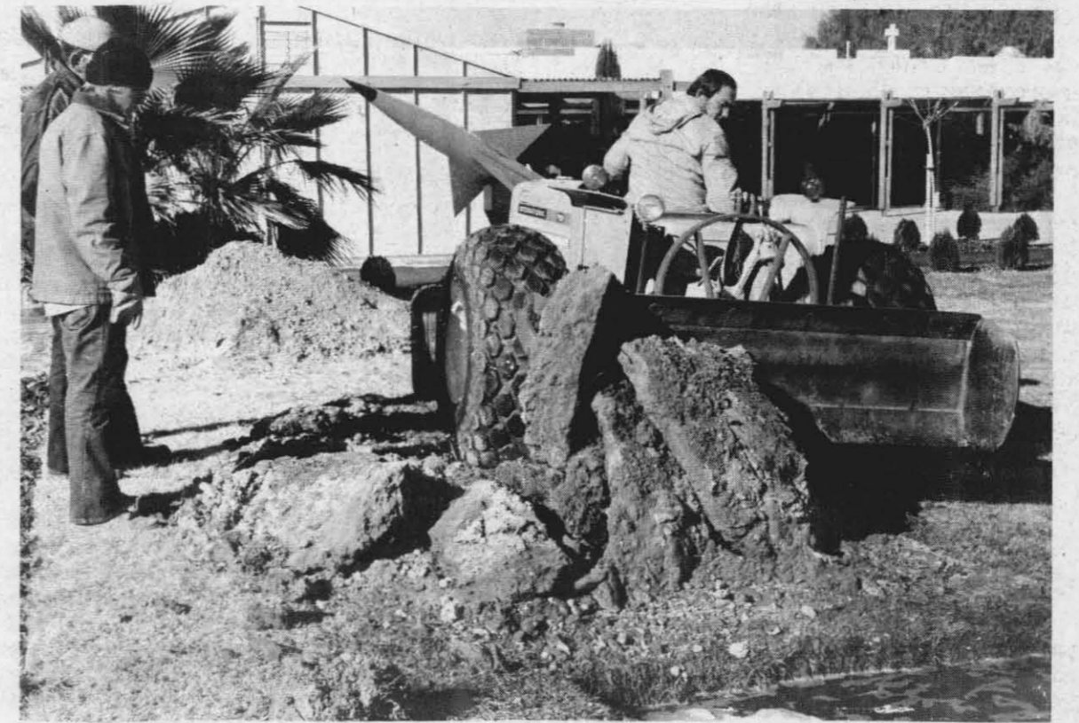
TRENCHING COMPLETED—Jim Lee, superintendent of the China Lake Golf Club, utilizes a tractor to fill a hole so that the trenching operation under way for the past three weeks at the golf course could be completed last Monday. The final 50 ft. of trenching on a job handled by the Automatic Irrigation Co. of Costa Mesa, Calif., was completed and work on replacing the main lines of the back nine irrigation system has begun. Bundled up for the extremely cold weather during the trenching operation are (at left) two employees of the firm owned by R. H. McCallum, of Costa Mesa. Work on the $40,000 contract was started the second week in November. —Photo by PH2 D. W. Yeatts
