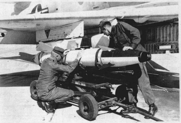
MARINES LOAD BULLDOG—Marines mount a Bulldog missile on an aircraft for flight testing on one of the ranges at the Naval Weapons Center. The Bulldog Weapon System, now in pilot production, was developed at NWC in response to the Marines' need for a close air support weapon. This laser-guided air launched missile provides first pass pinpoint accuracy in destroying surface targets.
