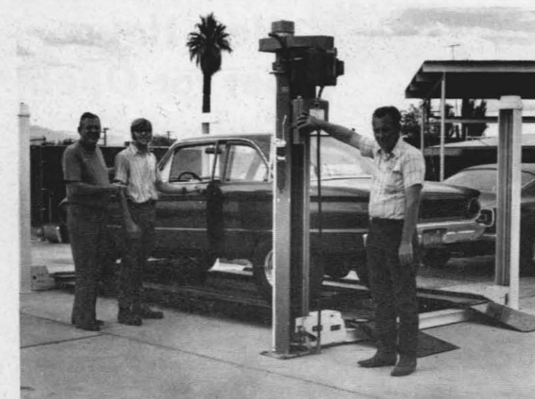
ELECTRIC HOIST INSTALLED — Military personnel and their dependents wishing to make use of the facilities at NWC's Auto Hobby Shop will now find their work eased by the recent installation of an electrically-operated hoist. Shown at the controls of the new hoist is Chief Richard Smith, manager of the Auto Hobby Shop, while Gabe Imer, head of Special Services, looks on as John Bitner, the shop's assistant manager, has his car elevated for a look at the vehicle's exhaust system. Before installation of the electric hoist, the west side of the outside parking area at the Auto Hobby Shop was resurfaced.
