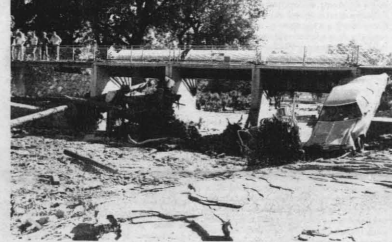
FLOOD DAMAGE—Debris, including a wrecked car swept against a bridge by the raging waters is typical of the damage left by the flood that devastated Rapid City, S.D., and neighboring communities on June 9. Weather expert Dr. Pierre St. Amand recently cooperated with two other internationally recognized authorities to complete a study on the flood and to make recommendations on ways to avoid such terrible destruction and loss of lives in the future.
