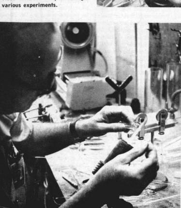
ABOVE, RIGHT-Griffith is seen working on another inner part of an AGILE detector package. Here the metal leads are being set in the glass to make the electrical connections for the detector, which will be mounted inside the glass. RIGHT—The Code 60 glassblower is seen working with one of the basic forms of many blown glass art forms. This is the body of a swan.
