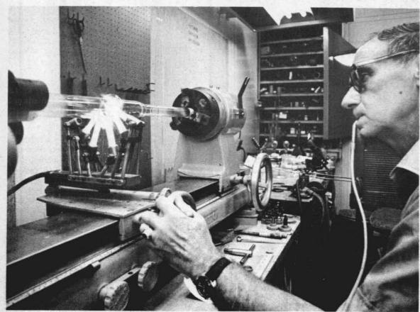
PRECISION WORK—Thomas Griffith, a glassblower in Code 60, heats glass tubing to form the second section of an expansion bellows. The section to the right of the burner has already been formed. Expansion bellows are used for thermal and shock isolators in glass apparatus. Griffith, who learned his glassblowing trade just after World War II, is a master of this ancient art.
