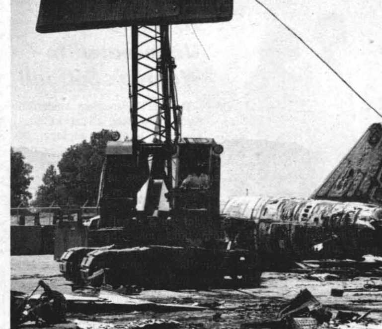
SALVAGE WORK UNDER WAY —A crew of workmen from the Artko Corp. of Tucson, Ariz., recently began the month-long task of salvaging metal from wrecked aircraft bodies that have been collected in a storage area at the Naval Weapons Center. A heavy, armor-plated blade that is lifted into the air by a huge crane is used to cut the airplane fuselages in half. It also is required as a part of the demilitarizing process that aircraft wings and tail sections be cut off and that the fuselage be split in two. The Tucson firm has a contract to pick up 500,000 lb. of wrecked aircraft. A 10-ton forklift is being used to load the scrap metal onto trucks that will transport the aircraft parts to a smelter. The end product of this effort will be aluminum ingots that sell for between 3 and 4 cents per pound. The wrecked aircraft that are being demolished have been used here as targets in testing a wide variety of missiles, rockets and bombs. —Photo by PH2 G. L. Taylor
