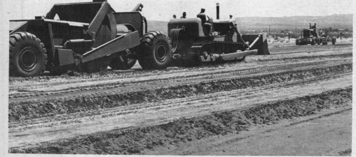
SEABEE RESERVES HELP OUT —A big assist was provided over the past weekend by more than a dozen SeaBee Reservists from Bakersfield, members of Sub-unit 11-21 of Mobile Construction Battalion 17. The SeaBees turned out to handle the job of grading a parking lot area at the site of a golf driving range and miniature golf course that is scheduled for development in Ridgecrest. The visiting SeaBees made good use of the heavy equipment made available to them by the Naval Weapons Center as they worked throughout the day on Saturday and from early morning until noon on Sunday. In addition to completing the parking lot grading work, the SeaBees also moved a building onto the site for use as a field office in connection with this Ridgecrest Improvement Committee project. The new community recreation area is being developed on a 19-acre parcel of city-owned land that is located just east of the fairgrounds in Ridgecrest.
