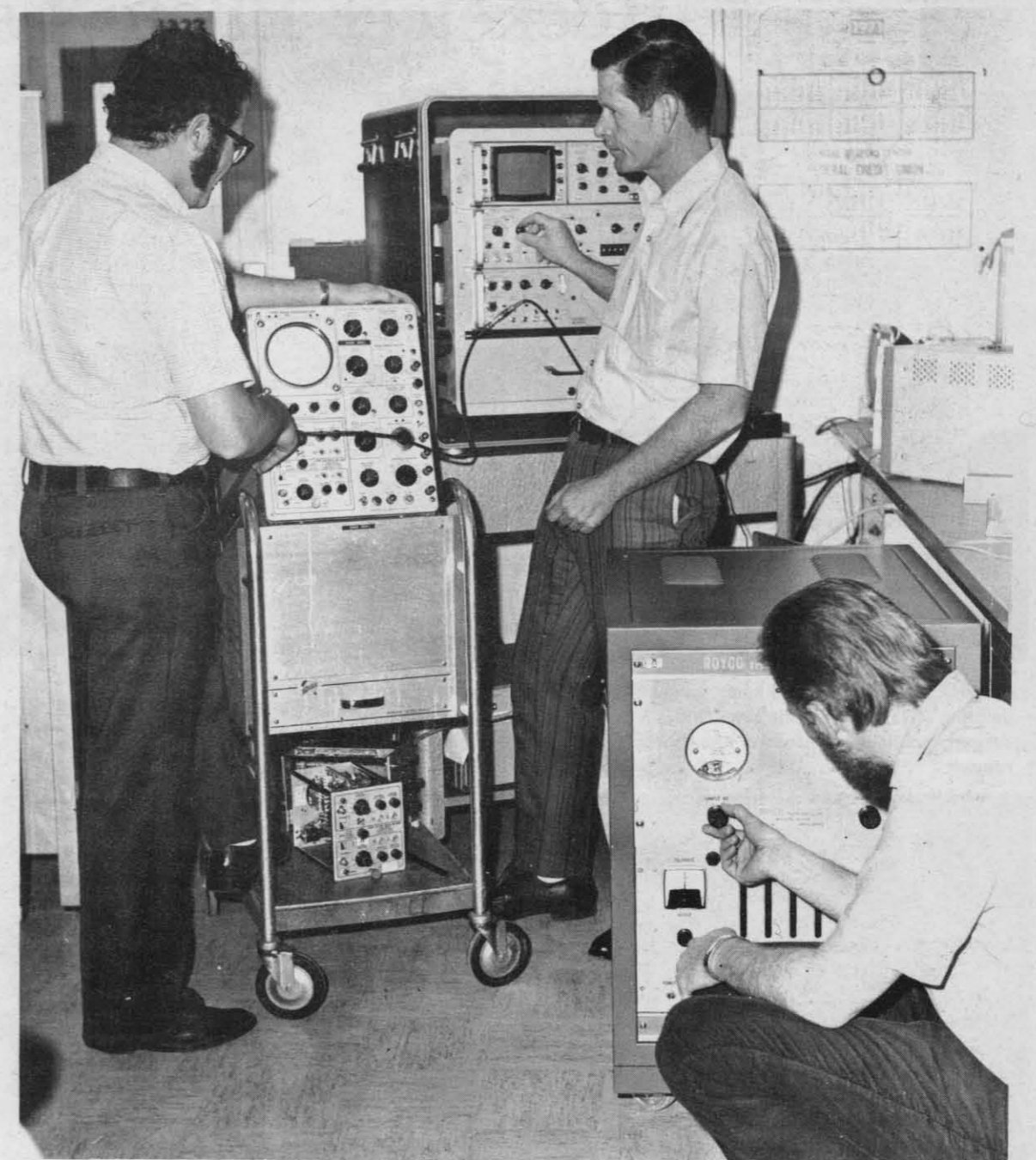
THREE MEMBERS OF the team set up a sampling run. From left to right they are Edward C. Ratto, a meteorologist, Walt Becktel, an electronics technician, and Paul Owens, a physicist. Ratto watches the oscilloscope to check interference patterns, while Becktel operates a multi-channel pulse-height analyzer. Owens is reading the particle analyzer which counts particles on the air that range from 3/10 microns to 10 microns.
