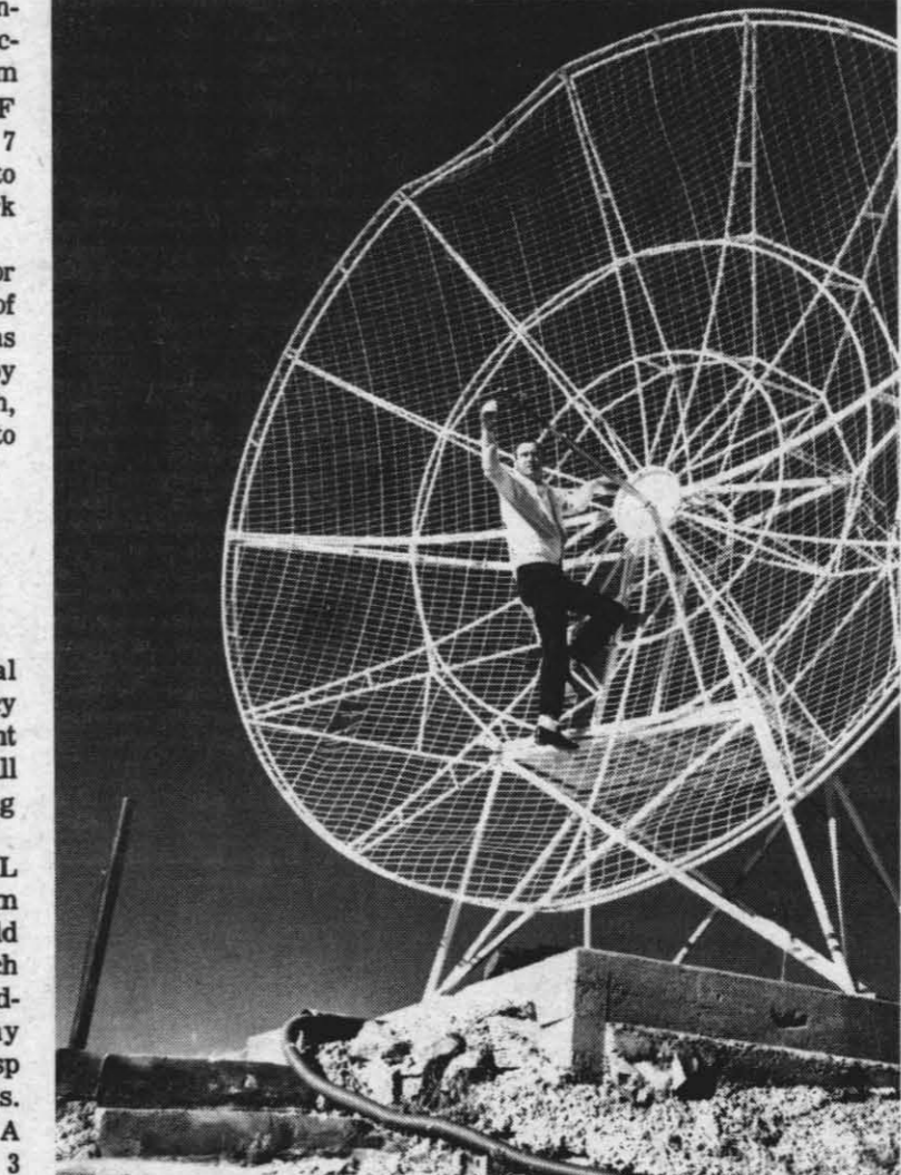
FINAL ADJUSTMENT MADE—Dick Furstenberg, who directs operation and maintenance of the TV booster station at Laurel Mt., checks over the large receiving antenna that has been installed to pick up the Channel 28 educational TV signal from Mt. Wilson.
