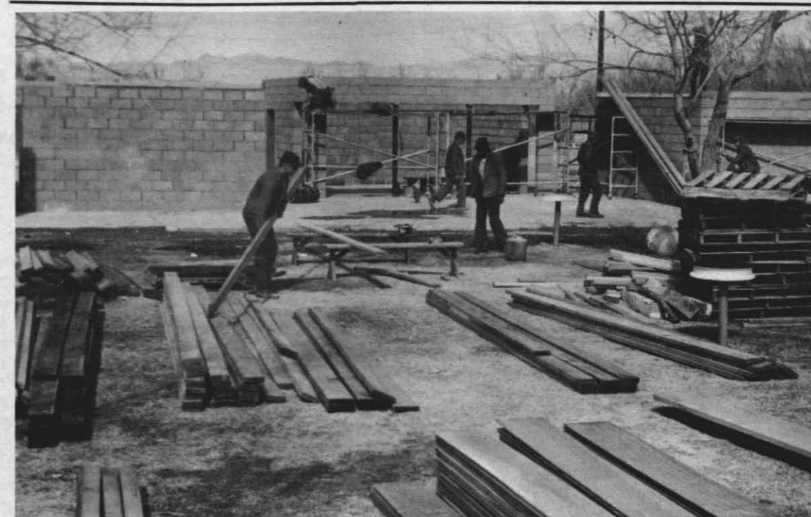
IMPROVEMENT WORK CONTINUES—Spearheaded by a handful of Sea Bees, who have been assigned here from Navy Construction Battalion 3 at Port Hueneme, and with the assistance of another eight or ten volunteers from among Naval Air Facility enlisted personnel, work is moving steadily ahead on improvements at the NAF swimming pool and recreation area. This project, part of the Navy's Self-Help Program, calls for the construction of a concrete block building that will house a snack bar in the center and be flanked by separate heads for men and women as well as showers equipped with hot water. The work, which is expected to be finished by the latter part of March, is now approximately 40 per cent complete, according to Ens. D. G. Morris, CEC, USNR, who is coordinating the activity. The new building will replace older, less permanent facilities at the NAF swimming pool.
