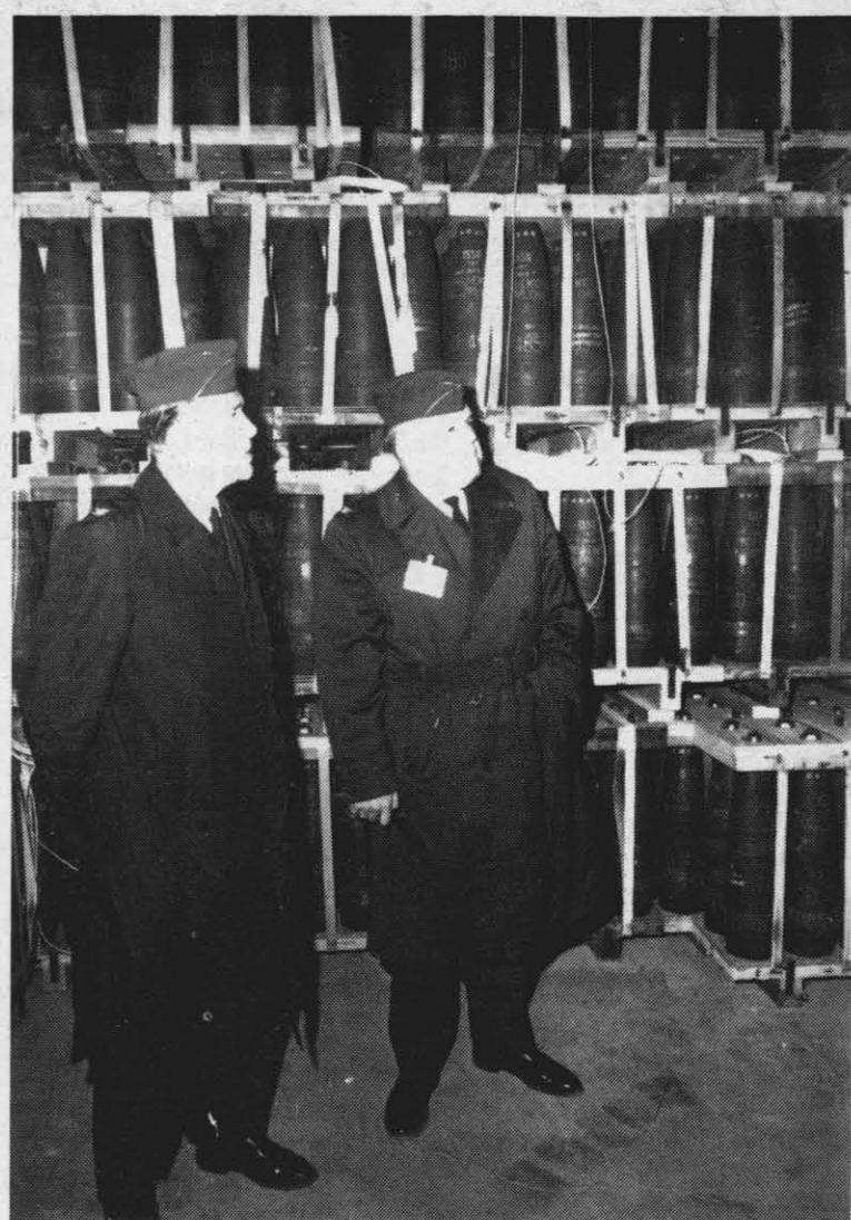
READY FOR BLAST —Some of the 13,700 155mm projectiles containing roughly 200,000 lb. of TNT that was exploded during the ESKIMO I test were inspected prior to the detonation by Col. William Cameron, III (at right), chairman of the Department of Defense Explosives Safety Board. With him is Col. W. K. Hillyer, from Headquarters, USAF, who is an alternate board member. The explosives were piled high within magazines located at the Randsburg Wash Test Range.
