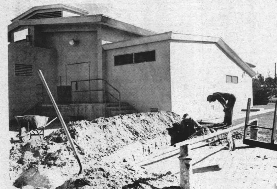
SCHOOL REHAB WORK PROGRESSES —Part of an extensive rehabilitation project at Richmond School calls for the lowering of existing pipelines carrying water and gas in order that some blacktopping work can be completed. Workmen involved in this task are employees of the Lockhart Plumbing Co., one of the sub-contractors on the job. Work on the renovation of Richmond School was commenced this past summer, and is expected to be completed by Christmas vacation time. After that, the contractor, the McKittrick Construction Co. of Los Angeles, will move his workmen to Vieweg School, where similar work is needed. In order to eliminate the need for classrooms at Richmond School this fall, a number of huts on the Murray and Groves School campuses were remodeled and put into use. When the rehabilitation work at Richmond School is completed, students assigned to it will vacate their huts, turning them over to youngsters from Vieweg School, who will have to leave their classrooms while the same kind of work needed at Richmond is being carried out at their school.
