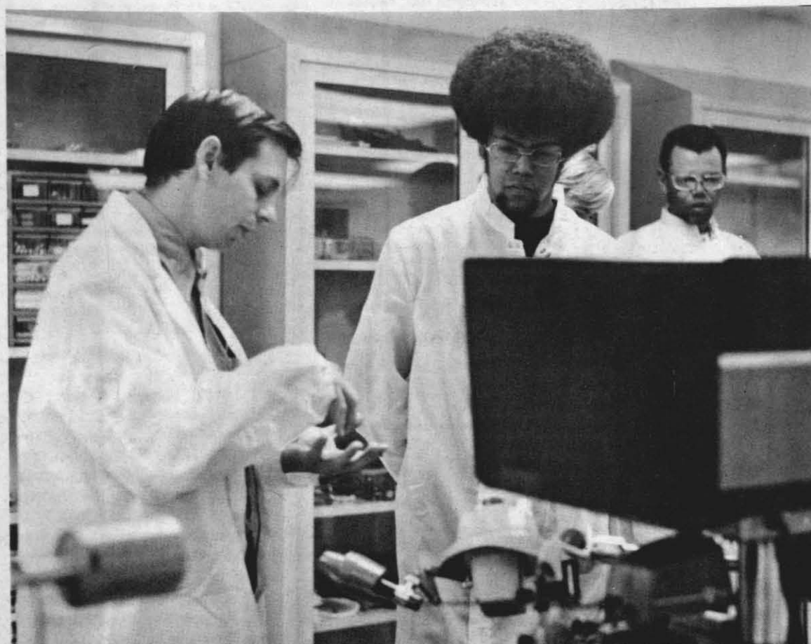
ABOVE -Dave Ritchie, (c), sophomore at Merritt College, Oakland, Calif., majoring in X-ray technology, learns about the different sub-miniature wire bonds as explained by Henry Blazek (l), while his father Milt Ritchie (r), looks on. Two types of bonding are Thermocompression and Ultrasonic welding and are both used to weld gold and aluminum wires to subminiature hybrid circuits.
