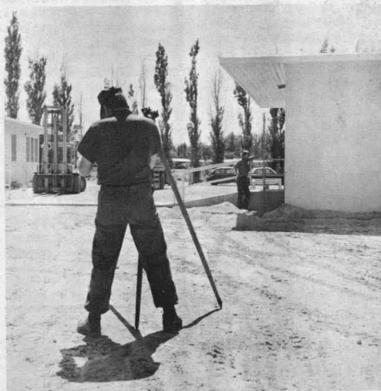
SEABEES LEND HAND -Work was started last Saturday by personnel of Mobile Construction Battalion 17, Sub Unit 11-2, on the development of a patio area between Wards 1 and 2 for the use of patients at the Naval Weapons Center Dispensary. The SeaBees will handle the final grading, install curbs, and later pour the concrete slab for the patio, in addition to putting in water lines and bubblers needed for irrigating the ground cover plants and bushes that will be planted by members of the Oasis Garden Club.
