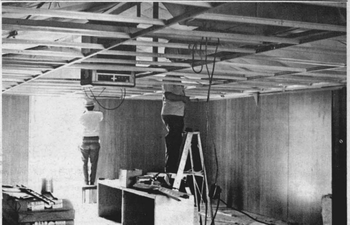
ELECTRICIANS RUSH to complete the wiring prior to finishing one of the huts on the Murray School campus. All of the huts (15 at Murray and 7 at Groves) have been completely renovated with new wiring, ceilings, carpeting, walls of rich-looking paneling and color-schemed blackboards.
