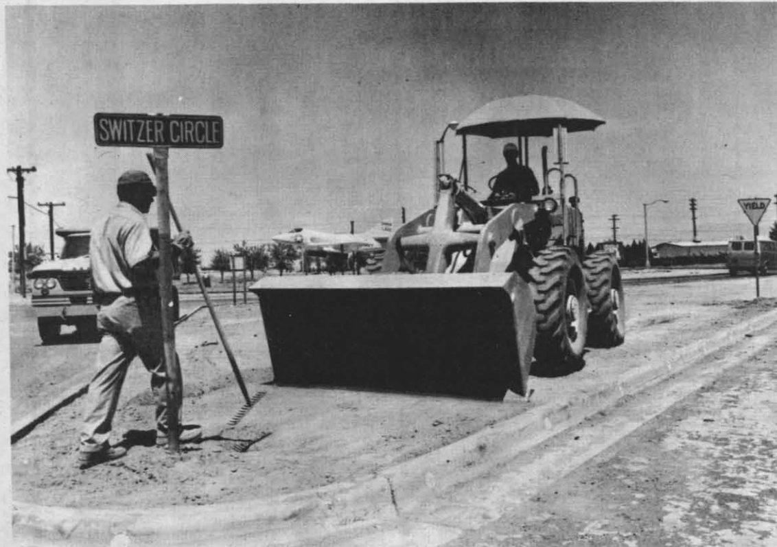
SWITZER CIRCLE REMODELED—Public Works workmen prepare Switzer Circle for a bed of rocks which will replace the grass on the islands and for a 30 foot radius on the circle itself. Surface and sub-surface damage from water to the road was the principal reason for the remodeling.
