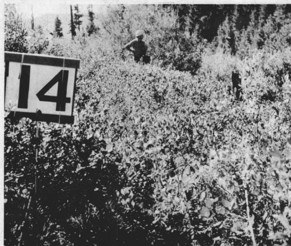
MISSOULA TESTS —Feasibility tests of the NWC-Forest Service fireline construction device conducted in August, 1970, at the Forest Service' Equipment Development Center at Missoula, Montana (MEDC) demonstrated that firelines could be constructed in
