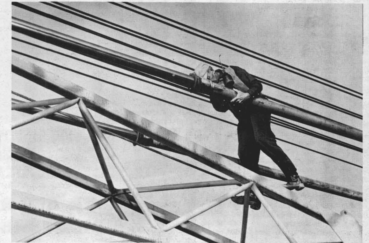
PERCHED HIGH above the ground, on precarious footing, LeRoy Printy routinely oils the seals on his crane. Much care is taken of all division equipment.
