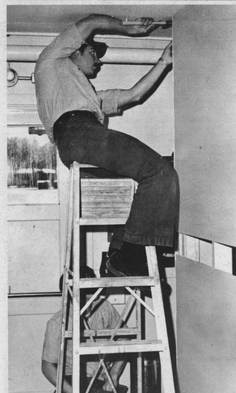
Z-GRAM IMPLEMENTED IN BARRACKS —An Clark (top of the ladder) and AOAN Stevens, enlisted personnel of the Naval Air Facility, are actively implementing Z-gram 22, which urges the use of a self-help program to improve shore establishment habitability. The sailors, with technical guidance from the Public Works Department, are in the process of converting cubicles into rooms in the lower deck of Barracks 3. Without the self-help program, such projects to improve living conditions for enlisted personnel stationed at NWC probably could not be accomplished, or would be unduly delayed.
