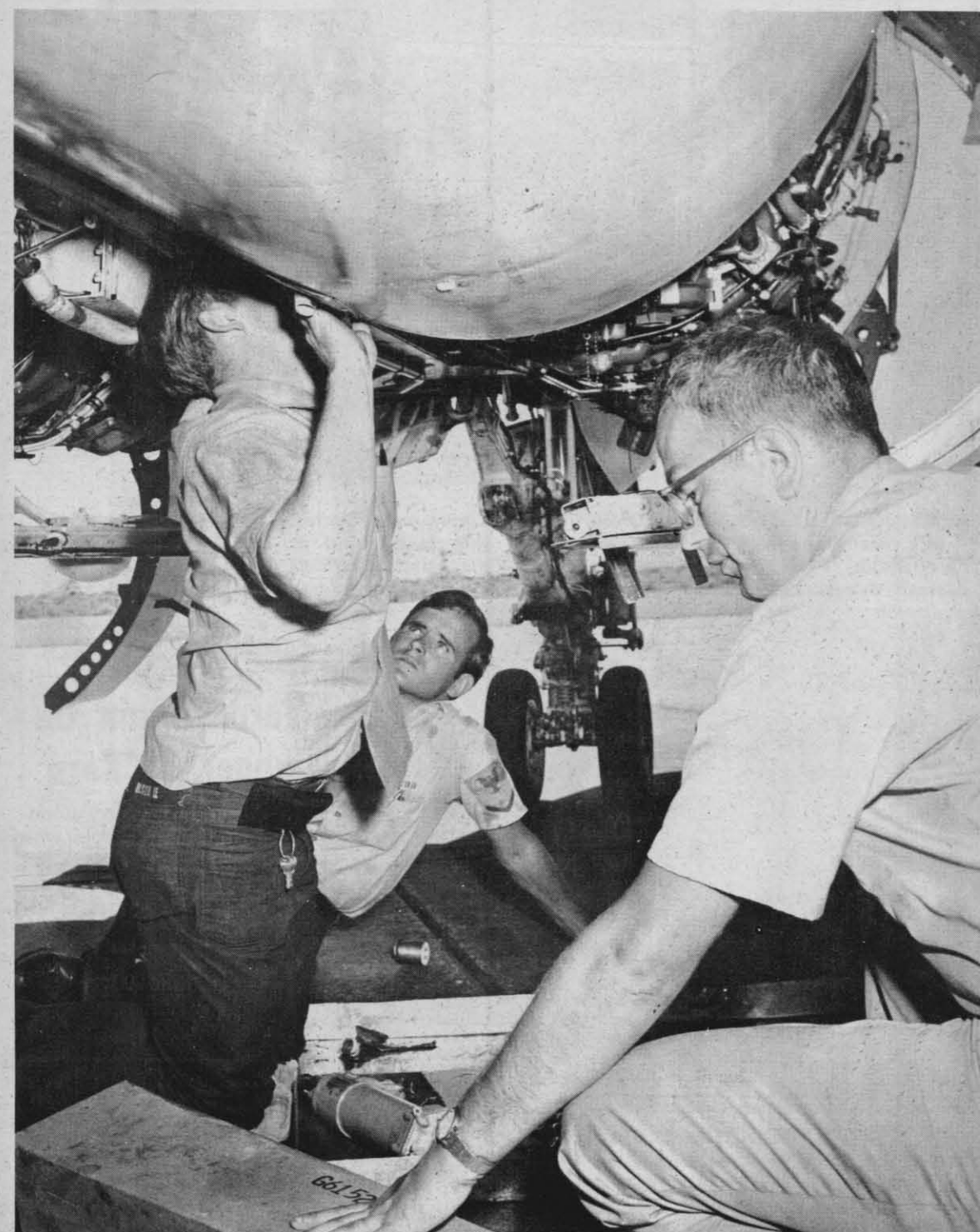
ATC DON MYERS (r) and ADJ3's Larry Olson (l), and Gary Webb of VX-5's Detachment at Oceana, Virginia, repair an engine on an A-6 Intruder. Det O has a complement of three A-6's and conducts tests of
