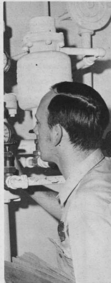
LT. PINNEY inspects a sprinkler system. Inspections of the sprinkler systems on the Center are done on a monthly basis.
