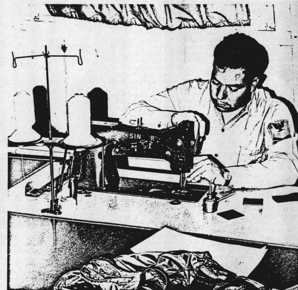
ABOVE — PR2 Robert Ruiz performs the daily maintenance necessary on the sewing machines used by the men in the Para Loft and Raft Shops to repair shrouds and raft equipment. BELOW — PR2 Don Gaines makes a check of oxygen mask regulator
