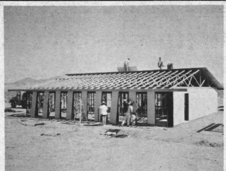
CLUBHOUSE NEARING COMPLETION—Members of the Sierra Desert Gun Club are shown hard at work as their clubhouse nears completion. All that remains is to complete the roof, add doors and windows and complete the inside work. The building includes an office, kitchen, rest rooms, club room and firing room. The new building is located adjacent to the NWC Security Police pistol range.
