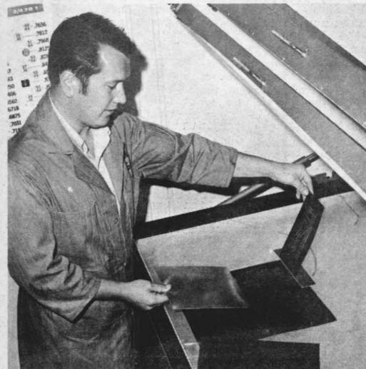
**PRINTING**—Charles Knowles prepares to print a circuit on a Micro-Miltronix double sided printer. The circuit is exposed to ultraviolet light from banks of lights above and below the board for a period determined by the timer in the foreground.
