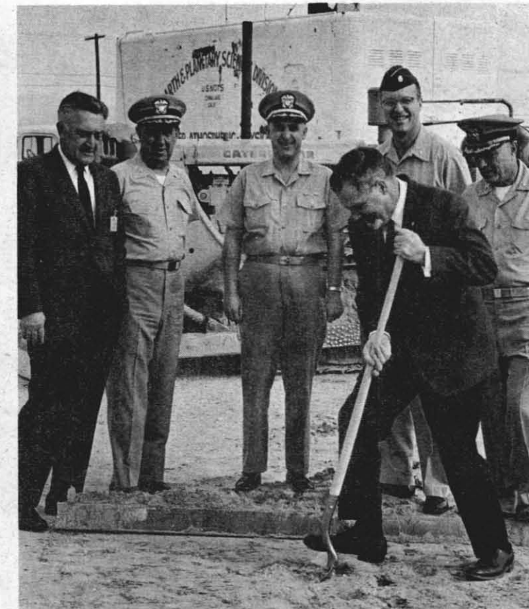
NEW QUARTERS PLANTED — Dr. Pierre St. Amand, Head of Code 60's Earth and Planetary Sciences Div. turns over the first earth on the side of the new laboratory-office building for the Joint Environmental Research Unit. The structure is to be completed soon, and will house about 100 people. Joining in the ceremony that took place in May, are (l-r) H. G. Wilson, Associate Technical Director; Capt. K. C. Abplanalp, Public Works Officer; Capt. Robert Williamson II, NWC Executive Officer; Air Force Maj. Ron Liningier; and Cdr. M. C. Jack, Division Military Assistant. The building will be adjacent to the new Warhead Building near Pole Line and Water Rds.
