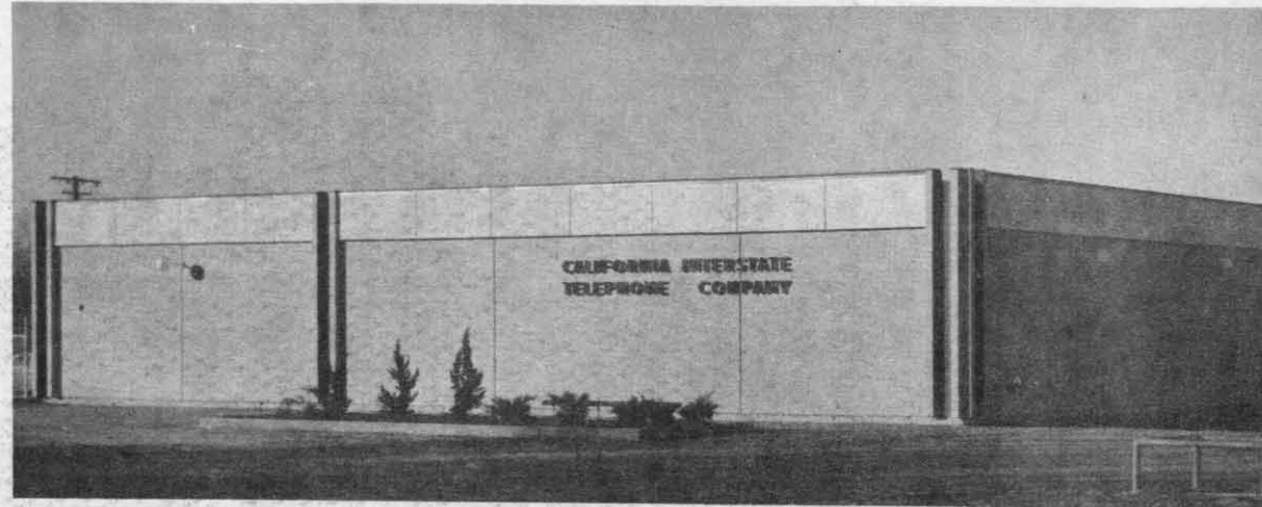
NEW TELEPHONE BUILDING — Construction has recently been completed on a new telephone facility that will serve as a switching center from some 2,300 stations on the base. Automatic switching equipment is now in the process of being installed. California Interstate hopes to start using the new equipment by August of 1969.
