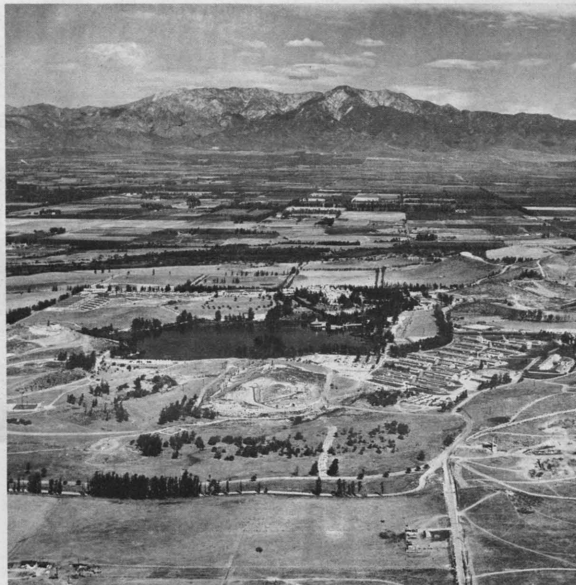
CORONA LABORATORIES — Aerial view shows complex of Corona Laboratories. In a regrouping of selected Navy laboratories into Centers in July, 1967, Corona became part of NWC. The Corona Laboratories employ approximately 1,000 personnel.
