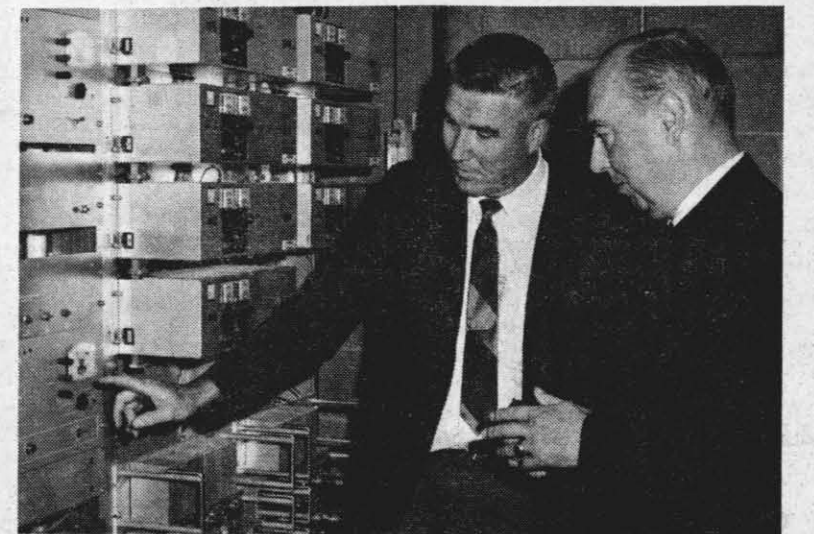
THE COMPLEX OF ELECTRONIC RECEIVERS, AMPLIFIERS, and other equipment required to operate the television translator facility atop "B" Mountain at the Center is explained by Hank Wair (left), Head of Metric Electronics Branch, Systems Development Department. The distinguished and interested visitor is George S. Smith, Head of the Broadcast Bureau, Federal Communications Commission Headquarters. They were accompanied on the tour by Capt. M. R. Etheridge, NWC Commander, and Smith's brother, Kenneth M. Smith, Mayor of Ridgecrest.
