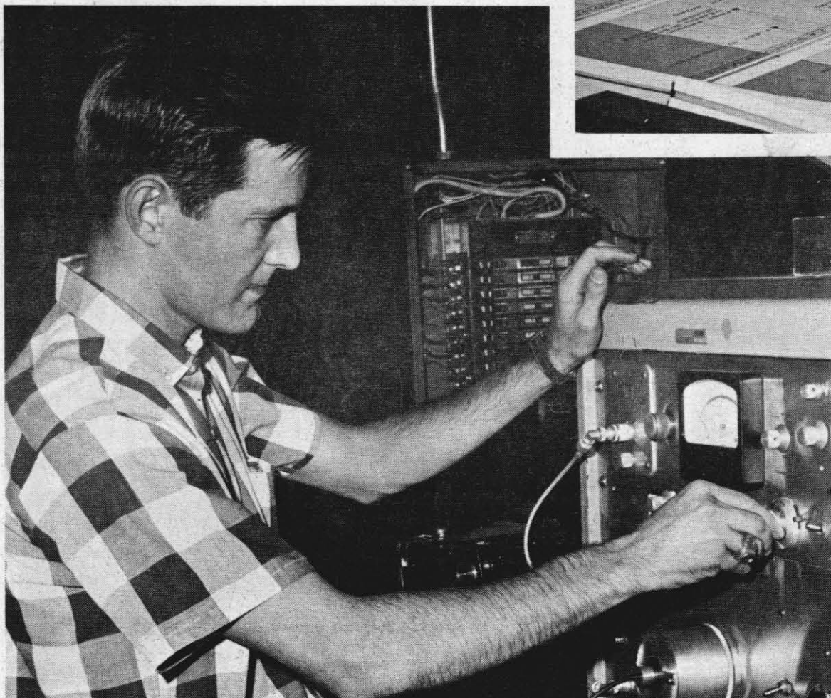
ROBERT SCOTT — Summer graduate student in Code 55, is shown checking out an interference filter he helped to design and build this summer for the purpose of locating pin holes in missile systems. Scott will be returning to the University of Oklahoma where he will work toward an advanced degree in physics.
