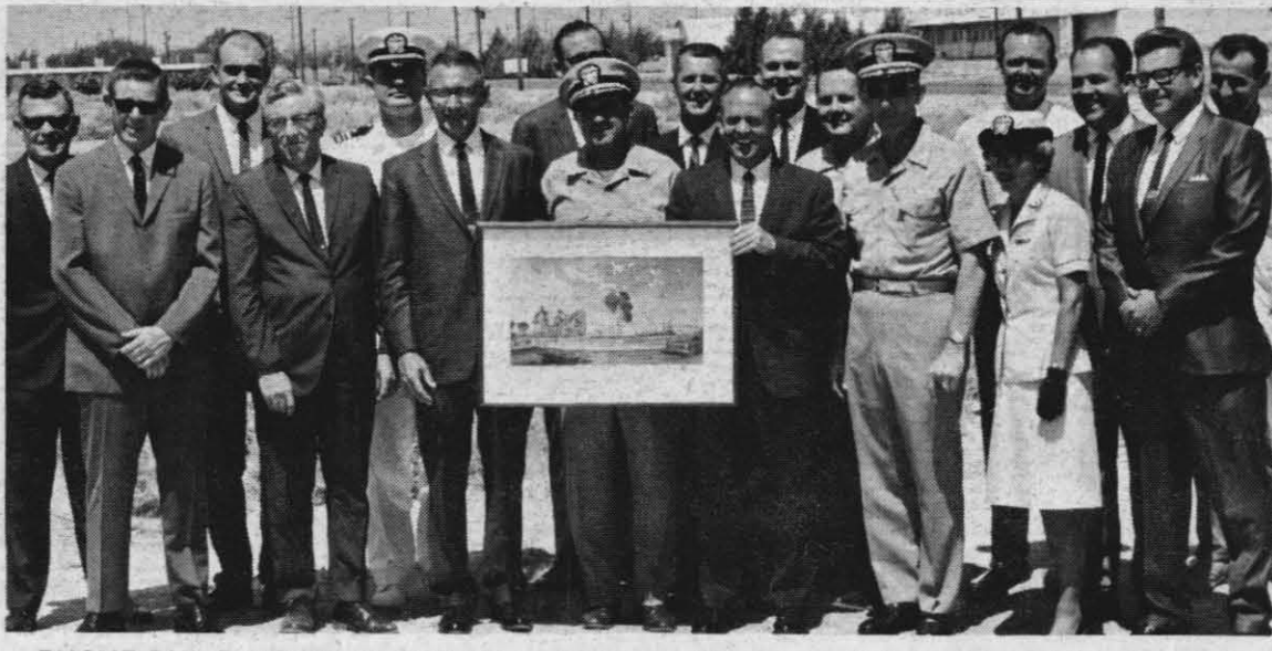
PHONE BUILDING TO RISE HERE — Capt. M. R. Etheridge, NWC Commander (r, center) is joined by California Interstate Telephone Co. and contractor people and other NWC officers as ground is broken for a new Interstate phone building. The company is expected to assume service for all residential phones in China Lake in late summer next year. Chief officials and NWC officers are (l-r) Bob Eddy (2nd from left), of the architects; Hal Hook (4th from left) of Hocker, Inc., Victorville; Lt. Col. John Loomis, Ass't. Public Works Officer (behind Hook); Capt. K. C. Abplanalp (center), Public Works Officer; C. N. Morris, Interstate's Vice-President in Charge of Operations; Capt. Etheridge, and Lt. I. R. Moore, Communications Officer.
