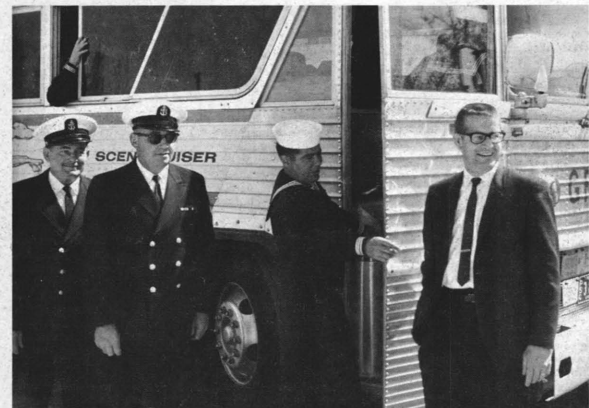
BUILDERS DEPART FOR GULFPORT — Their job is to help 700 other Reserve Seabees reactivate a naval station there—and to get invaluable training in such skills as timber towers and bridges, pile driving, poleline construction, well drilling, pontoon assembly, steel tanks and towers, water purification and asphalt paving. The 37 men of the local Reserve Construction Battalion Div. 1-2, led by LCdr. Carlton E. Hamel, S.C., USNR-R, were flown from Los Angeles to Gulfport.
