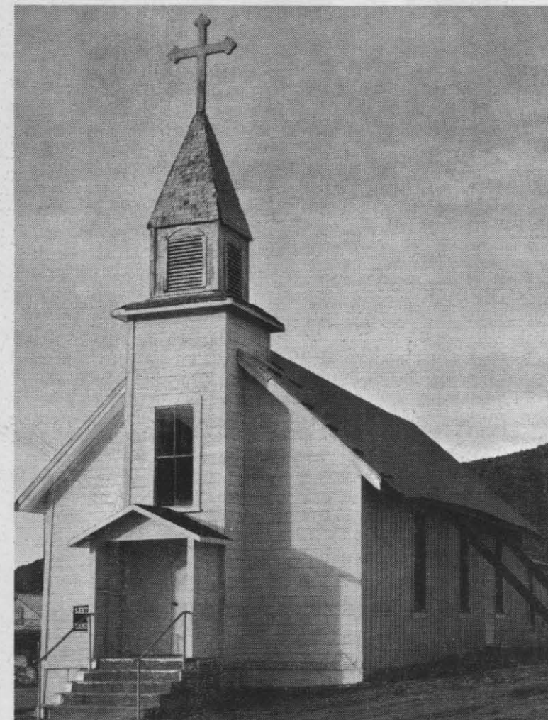
HISTORIC CHURCH — The Santa Barbara Church, located on the main street in Randsburg still holds regular services for the local population. Note reinforcing at side.
