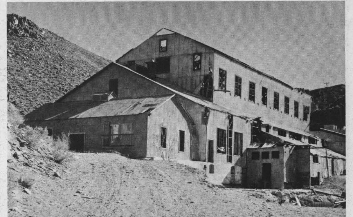
SILENT SENTINEL — Like a silent sentinel was, in its heyday, an elaborate facility of a long-gone, exciting past, the giant mill and engine room at the Yellow Aster Mine with gold filigree design still to be seen in the spokes of the steam engines flywheel.
