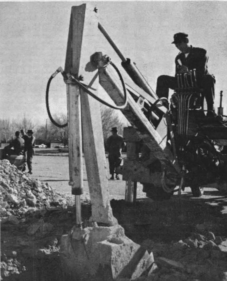
SURE HAND — Seabee reservist EOC J. Cashero from Bakersfield shows a sure hand in making excavation "on dotted line" at new playground along S. Knox Rd. between Renshaw and Randolph Sts. Much needed play area will have a fence along heavily traveled S. Knox and a complete sprinkler system to keep grass carpet green.
