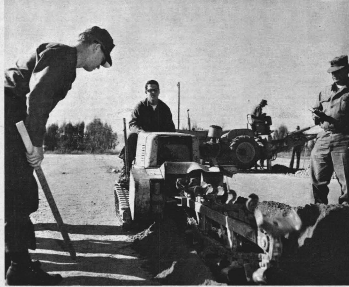
DIGGING PIPE TRENCH — Bakersfield Seabee CMA-2 Lynn Weeks operates trench digger on site of future playground while Cdr. W. G. Catlin and EOC G. L. Lantz check progress. The trench will contain sprinkler system pipes.
