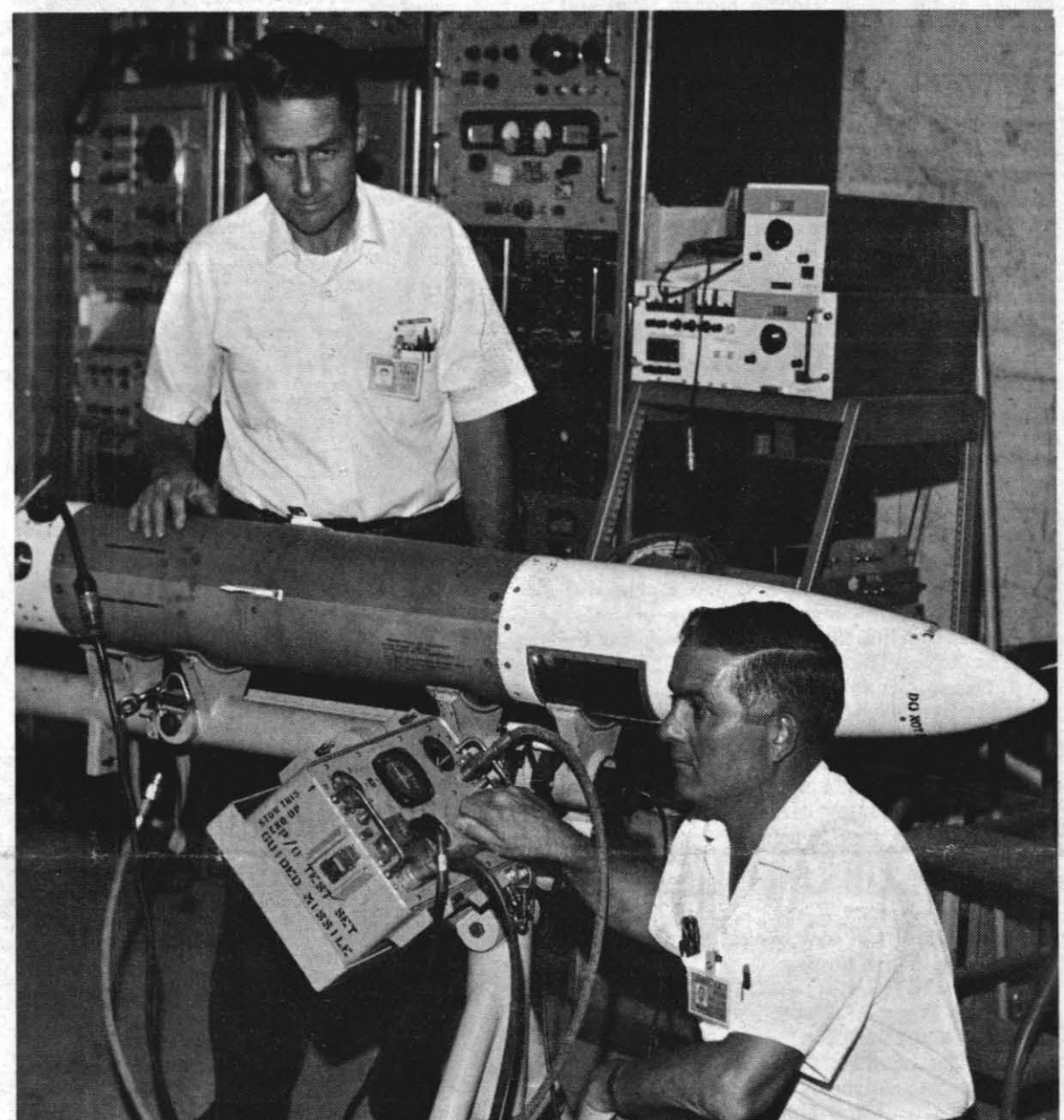
CHECKING OUT SHRIKE'S UHF — George Hudson, project engineer for the Shrike telemetry changeover from VHF to UHF, stands over a test bird while Monsie Stanley, electronic technician, checks a circuit. Stanley did environmental testing of the new ultra-high frequency components, which exceeded Shrike specifications. Both men
