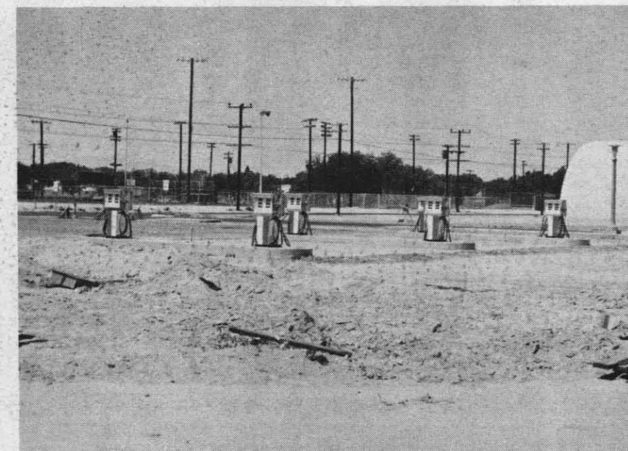
SERVICE STATION rises at shopping center; FEDCO will operate it.
