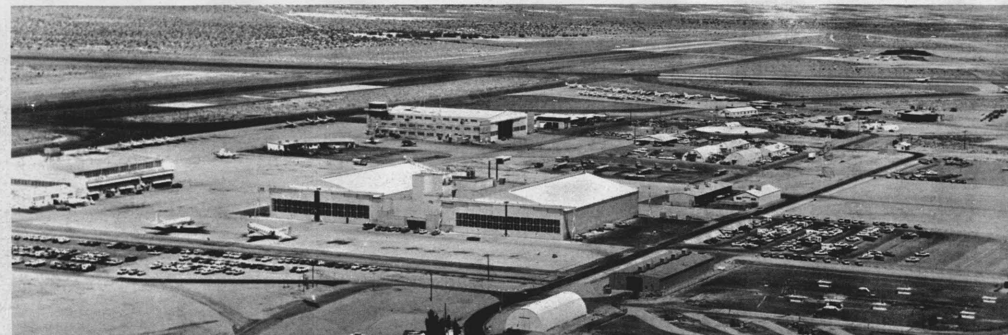
IDEAS PROVEN HERE —At NAF and VX-5 complex, new ordnance is proven; delivery techniques developed.
