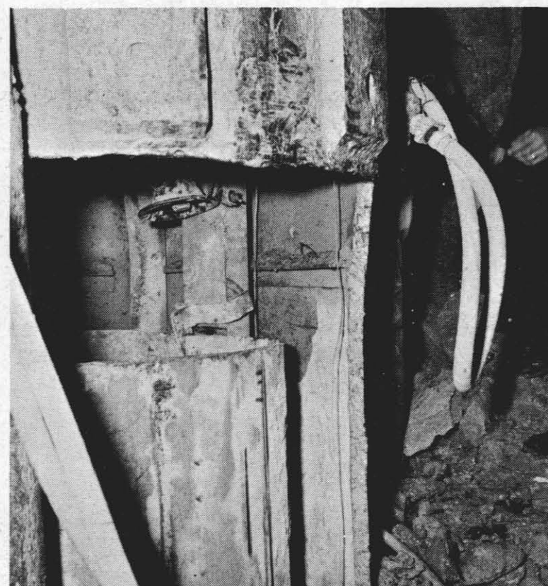
EXIT AT THE BOTTOM—Workers broke out of shaft bottom with a cutting torch. The small ports in strengthening structures above the opening allow worker to drill outward to test for water seepage. If necessary, grouting cement can be pumped through a valve to consolidate the rock.
